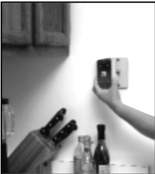
Remove phone and install filter on existing phone jack
